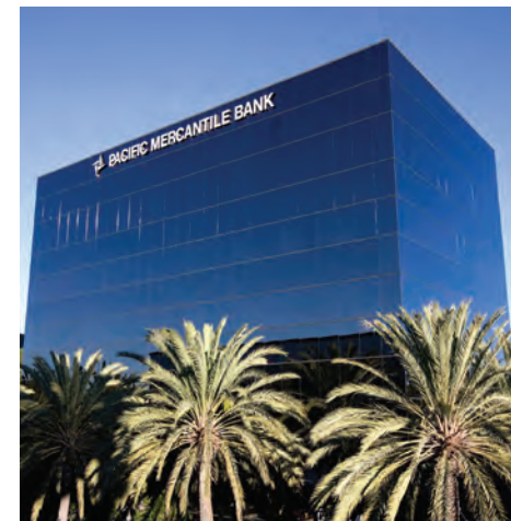
949 S. Coast Drive: headquarters of Pacific Mercantile, the seventh biggest OC-based bank by assets
