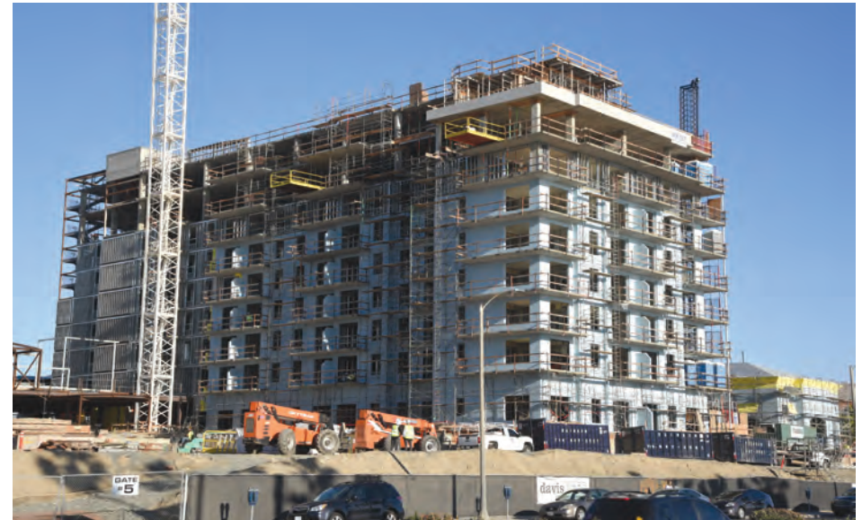
Add-on: under-construction Waterfront Beach Resort tower earlier this year
