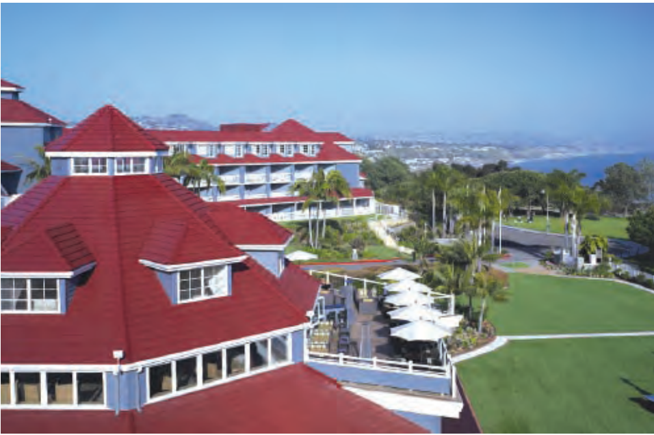
Spectacular coastal view of Dana Point from the newly renovated Laguna Cliffs Marriott Resort & Spa.
